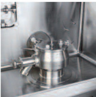
Detail Isolator Installation.
